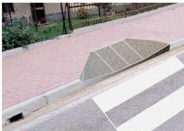
**RACCORDI PER MARCIAPIEDI E PICCOLI DISLIVELLI****1.3****SCIVOLO RETTILINEO CON DOPPIA RAMPA A PIANO INCLINATO.**
