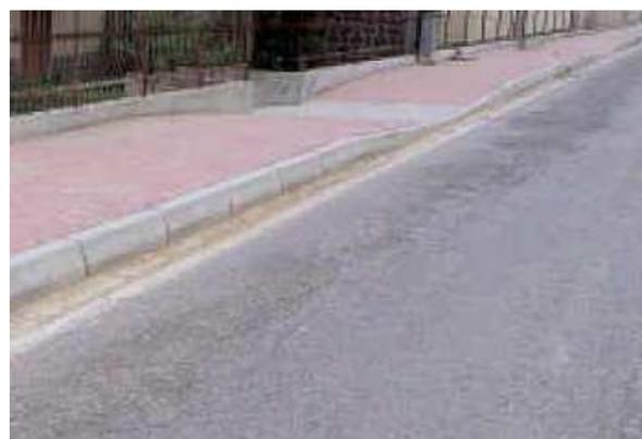
**RACCORDI PER MARCIAPIEDI E PICCOLI DISLIVELLI****1.4****SCIVOLO RETTILINEO CON RAMPE A PIANO INCLINATO POSTE ORTOGONALMENTE.**
